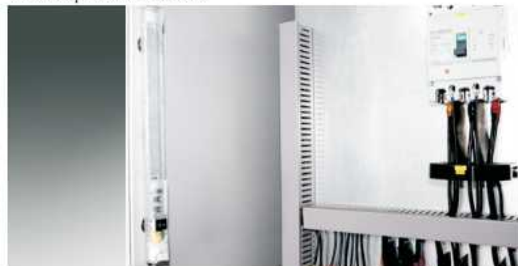
The side installation
